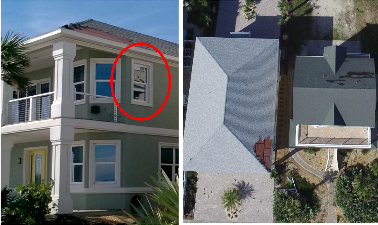
Figure 20: Ground view of broken window at 1424 S Ocean Shore Blvd (a) and aerial view of home with broken window and adjacent home which lost roof shingles (b).
